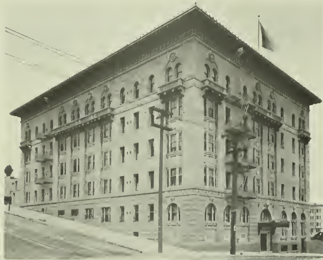
ST. DOMINIC APARTMENTS. F. H. Meyer, Architect.
